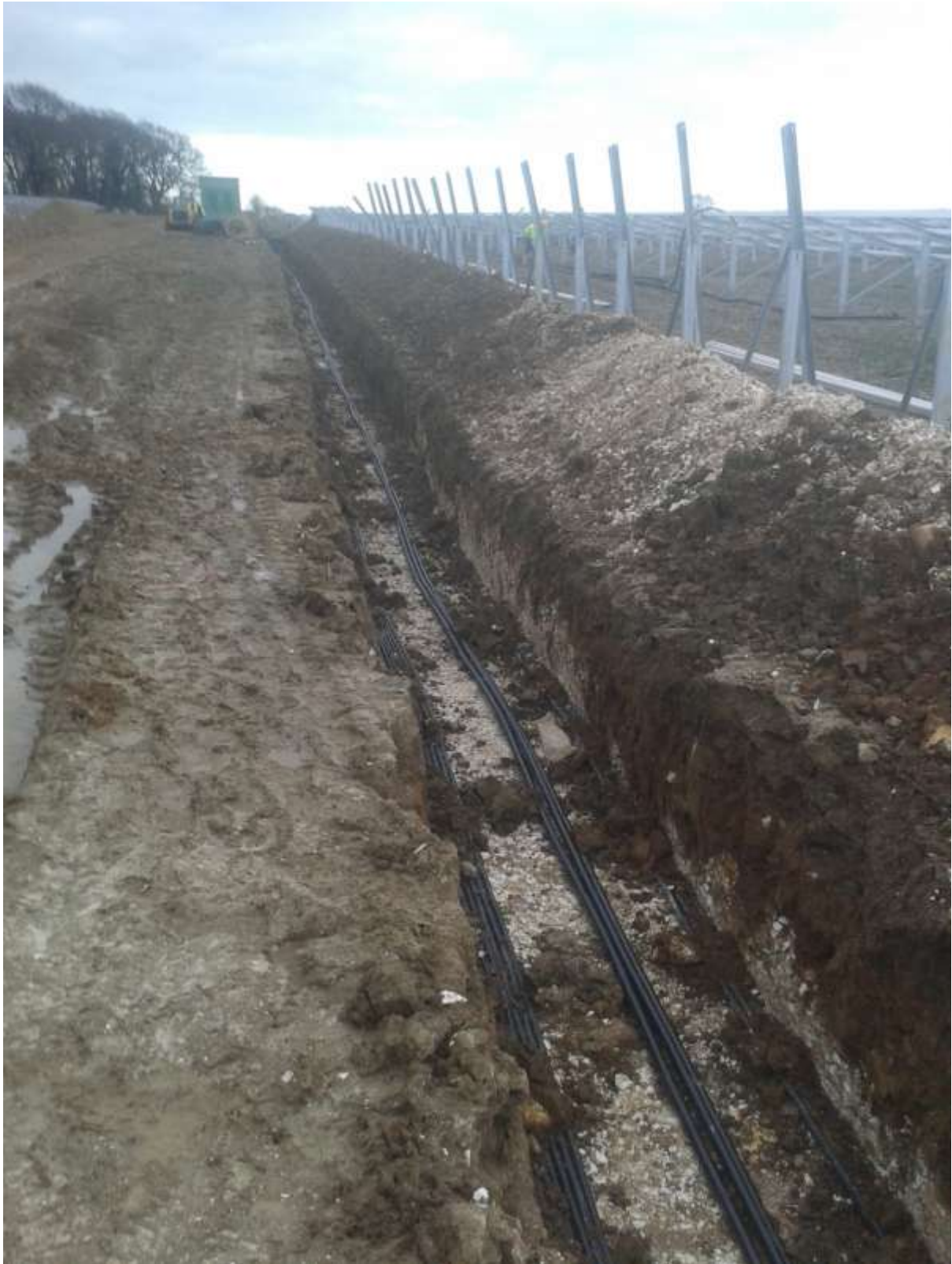
Plate 5. Cable runs to inverter (looking north-east)
