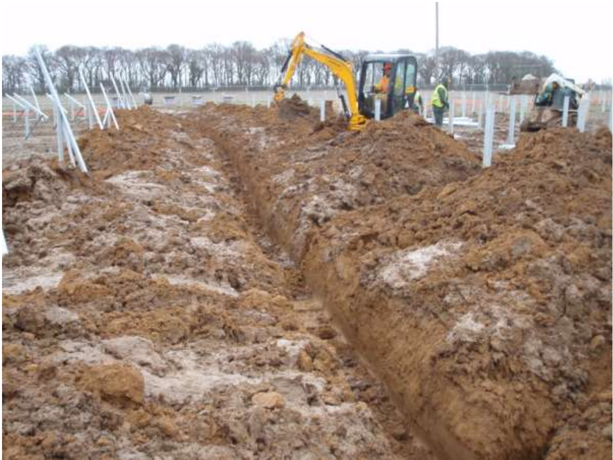
Plate 6. Spur trenches under construction (looking north).
