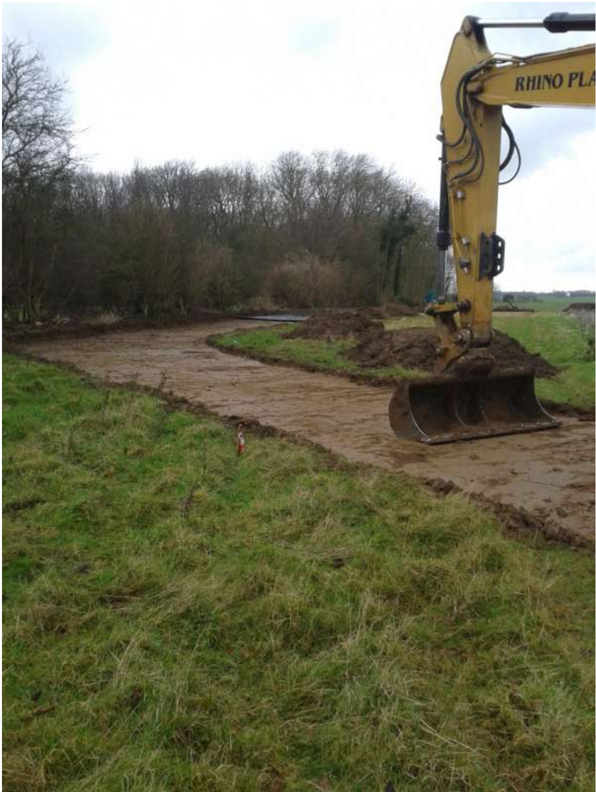
Plate 2. Access road being built (looking south-west)
