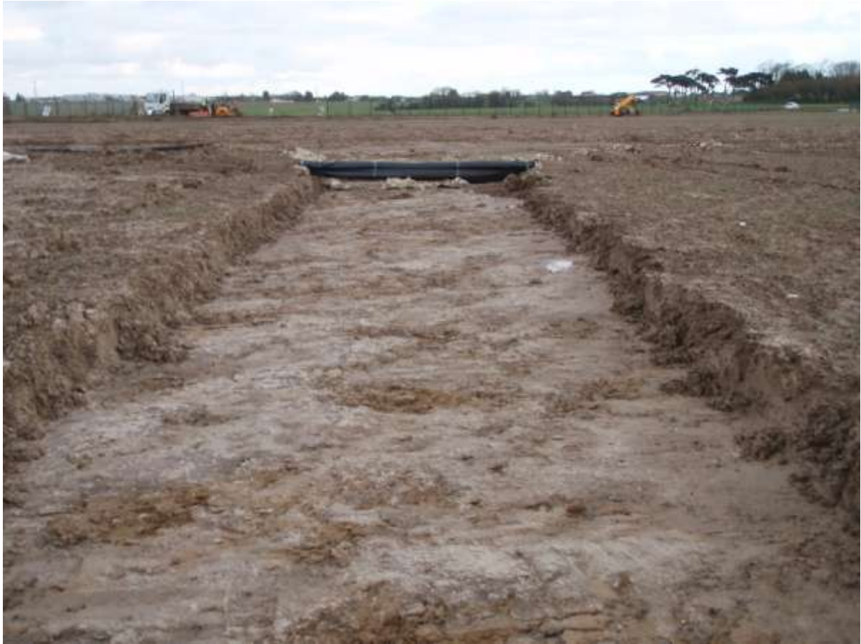
Plate 4. Construction of access tracks (looking east)
